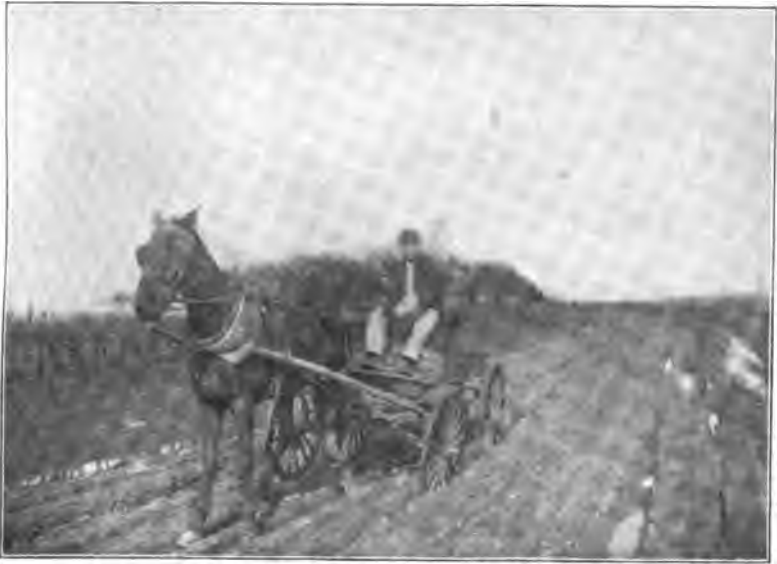
Neshanic road, Somerset Co., before improvement.
